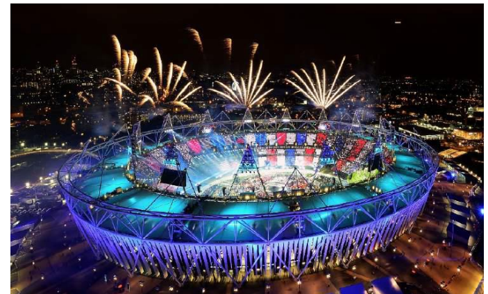
London Olympic Stadium, UK Buro Happold, 2012
