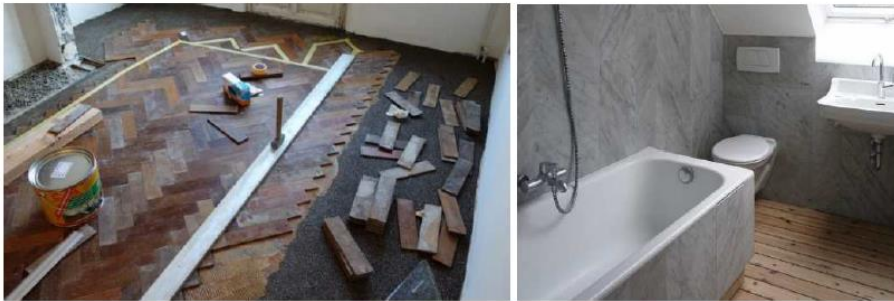
Figure 2. Warland - Incoming reclaimed materials: wooden flooring and marble
