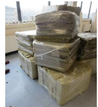
Figure 4. Horta-ONSS – repackaging of insulation for off-site reuse.
