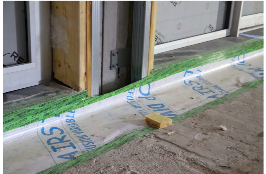
Air-tightening (© VUB Architectural Engineering)
