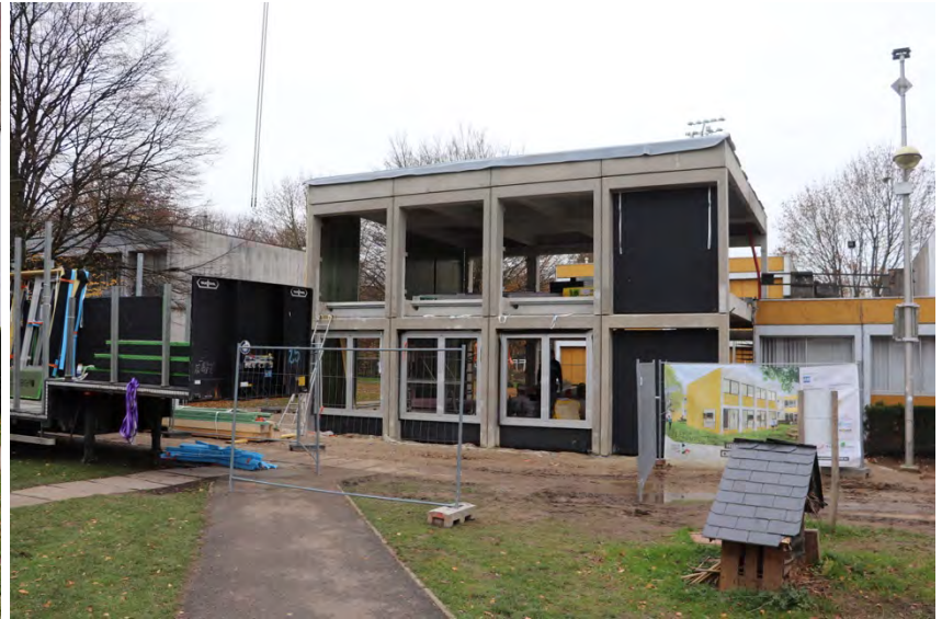
Installation of the façade elements (© VUB Architectural Engineering)
