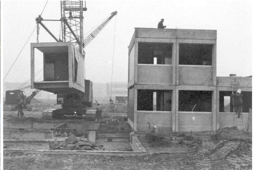
Installation of the Variel modules, 1973 (© Archive Technical Service, VUB)
