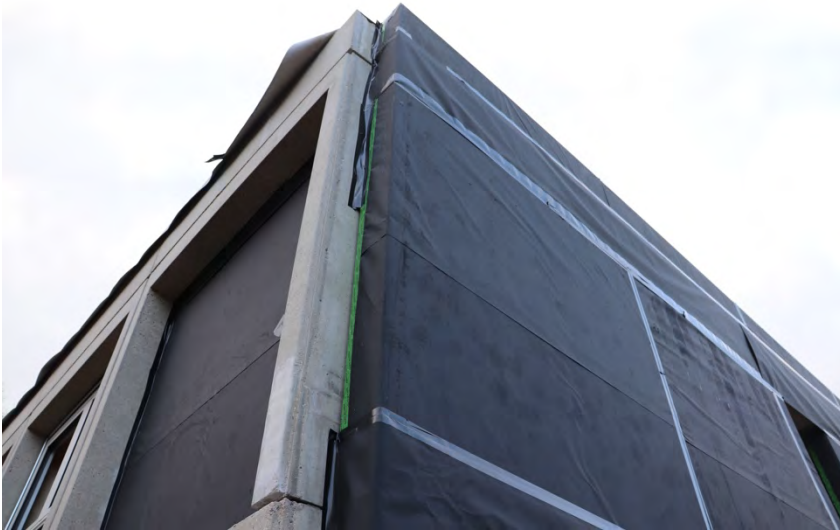
Waterproofing of the envelope (© VUB Architectural Engineering)
