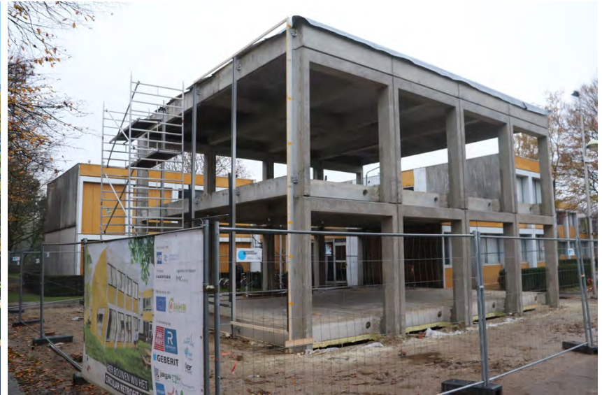
Stripped and sanded structure (© VUB Architectural Engineering)
