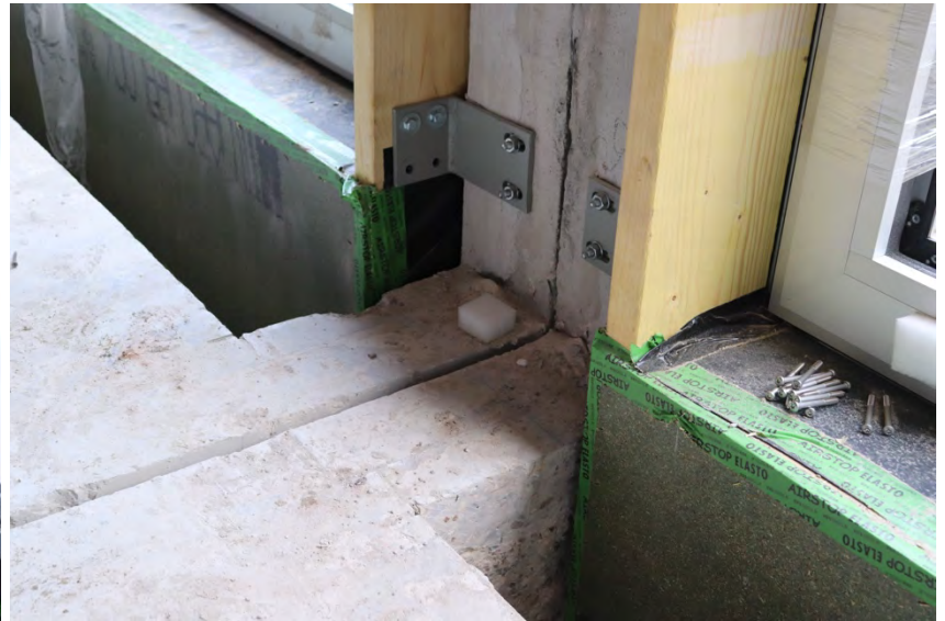
Connections of the façade elements (© VUB Architectural Engineering)
