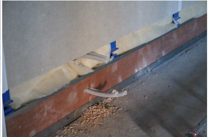
Services integrated behind removable plinth (© VUB Architectural Engineering)
