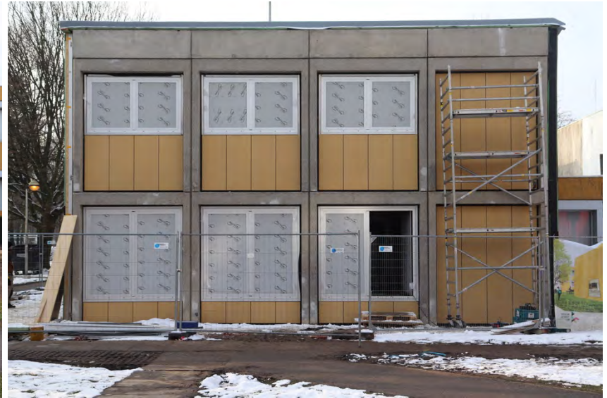
Installation of the cladding (© VUB Architectural Engineering)
