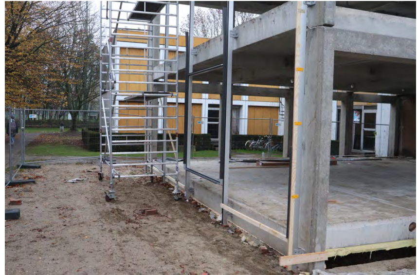
Construction of curtain wall (© VUB Architectural Engineering)
