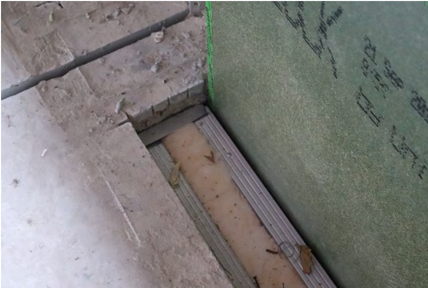
Insulation of cavities to ensure performance of envelope (© VUB Architectural Engineering)
