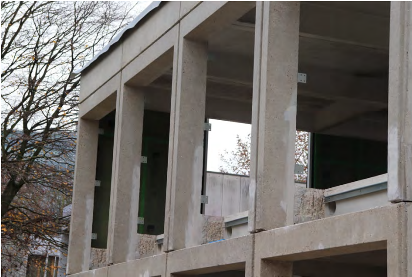
Connections for the façades (© VUB Architectural Engineering)
