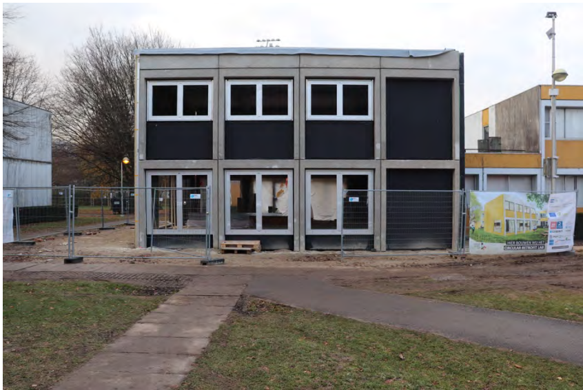
Installed façade elements (© VUB Architectural Engineering)
