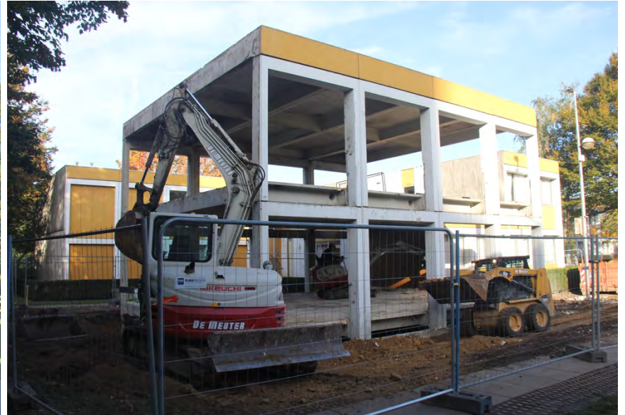
Partial demolition, stripping of eight modules (© VUB Architectural Engineering)
