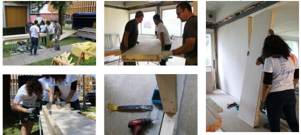
Figure 20: Construction of the Saint-Gobain P2 system, based on pre-assembled wall elements with a wooden structure
