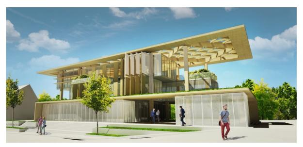
*Figure 5: GTB Lab transformation scenarios. The maximum scenario imagines the addition of two extra floors to the initial module . Half of the ground floor module can be disassembled and reused on the upper floors.*
