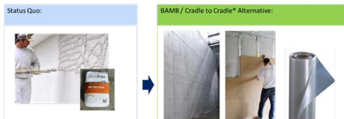
Fig. 10: Uncoated concrete walls facilitate their future potential recycling
