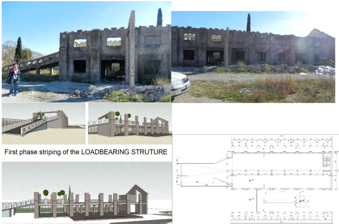
Figure 15: Representation of the existing building structure and the image of the building after removing all infill elements (non-structural elements).
